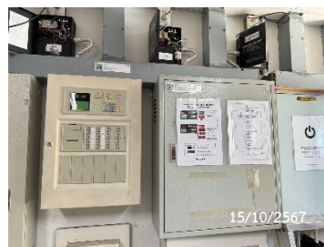
Fire Alarm Control Panel
